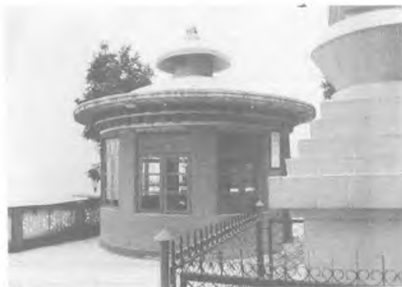
Plate 7 Lamp Hall (gSas-mkhar li-li bang-bang) (S. Yamaguchi, November 1998)
