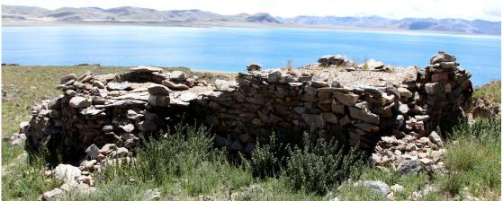
Fig. 1: The exterior of a smaller corbelled building that has retained much of its all-stone roof, located on the insular site of Do Drilbu (Do dril bu).
