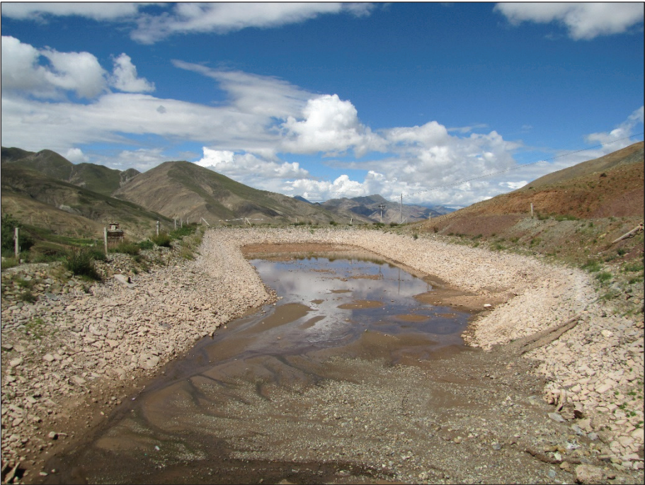
Plate 36 Bla rdzing (after the construction of the new road), 2016; Photo by JH
