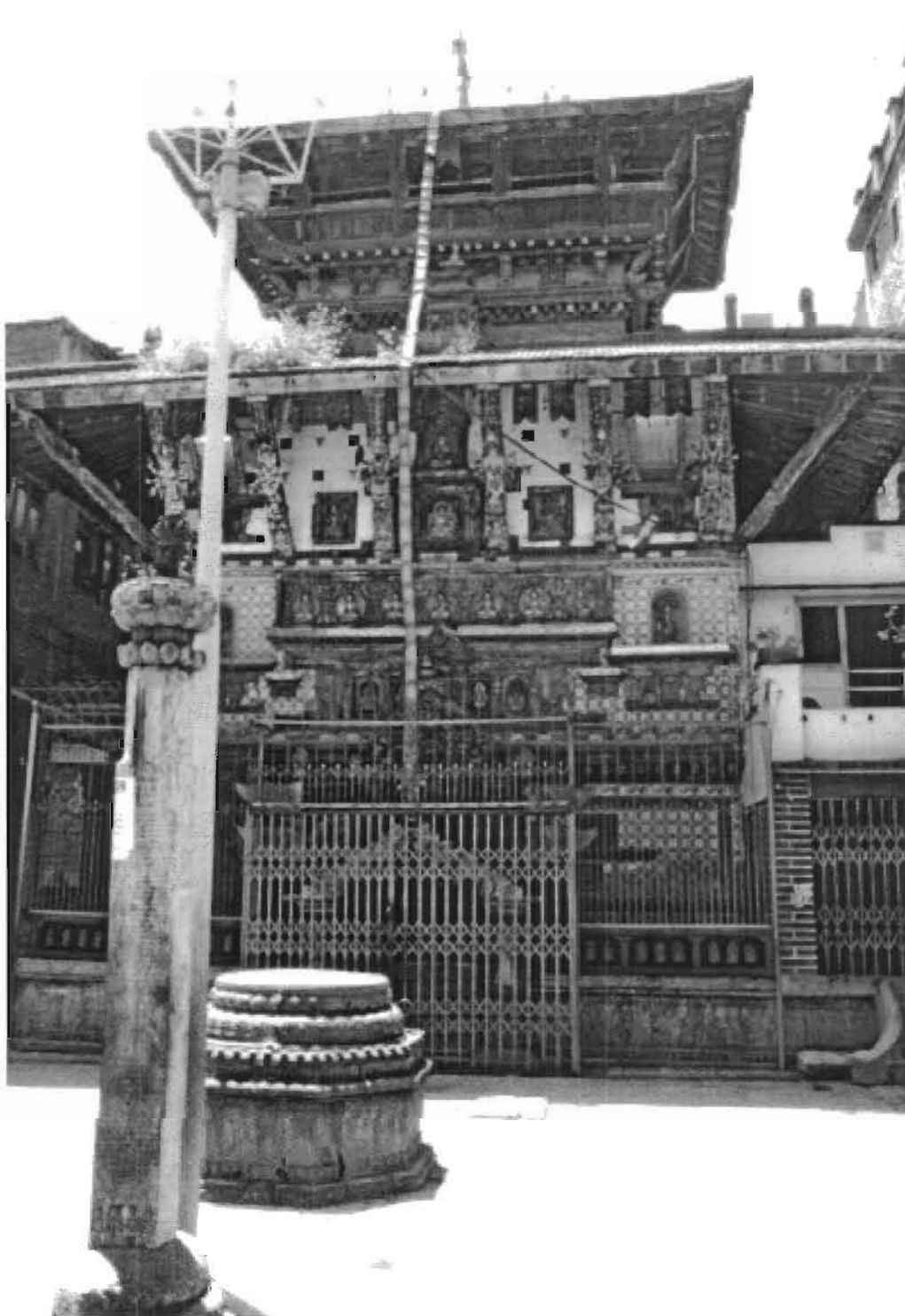
Figure 5.30. Interior Courtyard. Bu Bāhā, Patan. View of South Shrine Wall.
