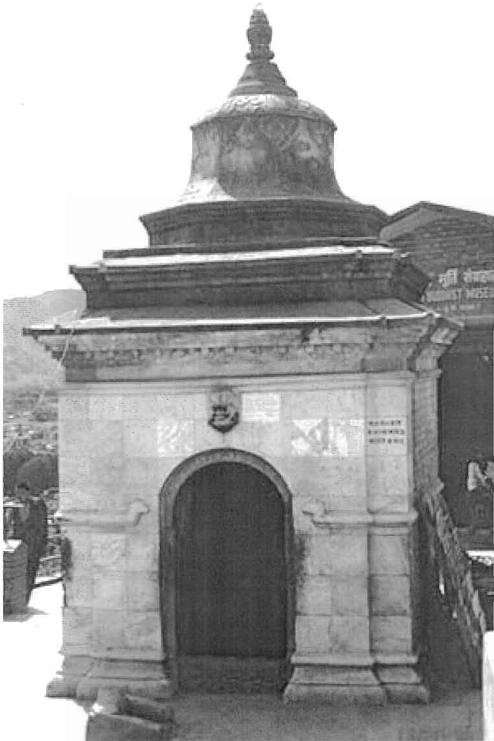
Figure 4.32. Vāyupur. Southwest side of Mahācaitya. View of east face.
