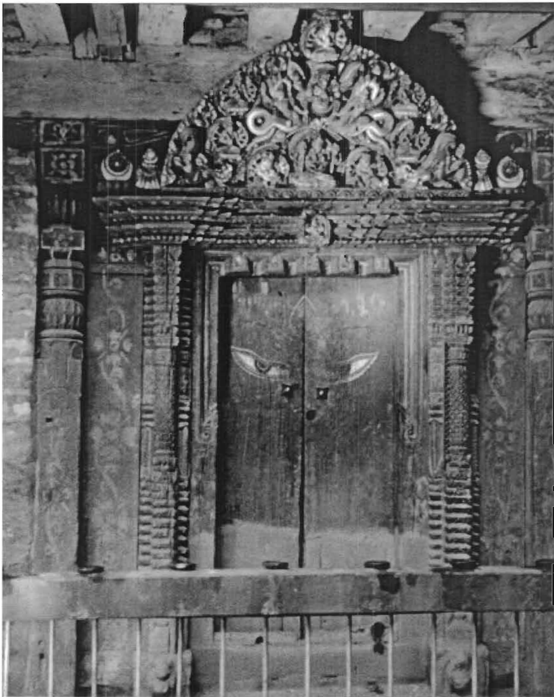
Figure 6.14. Door leading to āgam shrine. North courtyard wall. East end. Gujī Bāhā, Patan.
