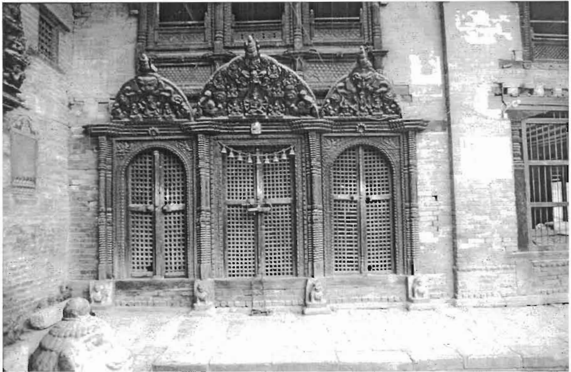
Figure 5.53. Exterior of Vajrasattva shrine. West courtyard Wall. Ha Bāhā
