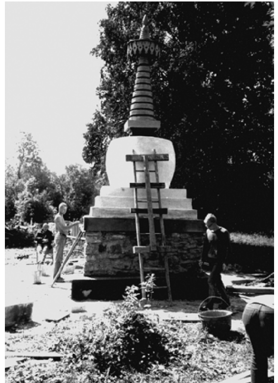
Building the first stupa in Läänemaa
